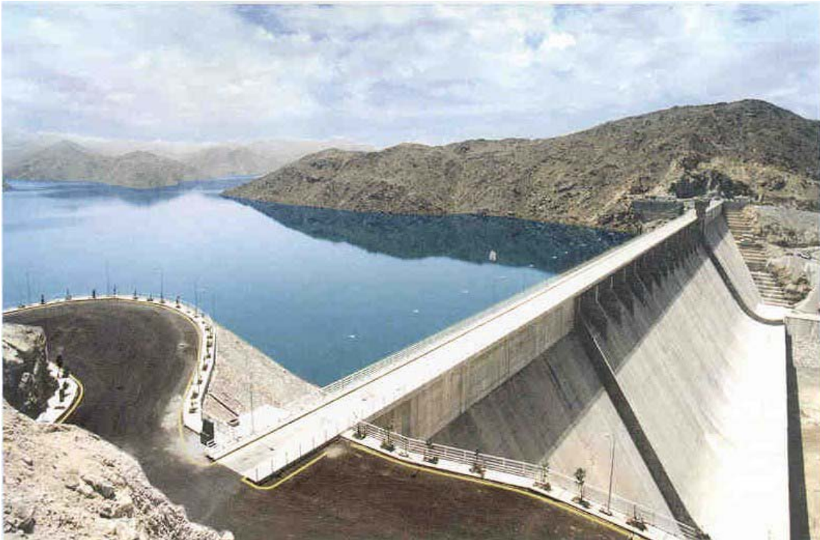
Figure 11a: Selected Pictures of Some Saudi Water Dams
