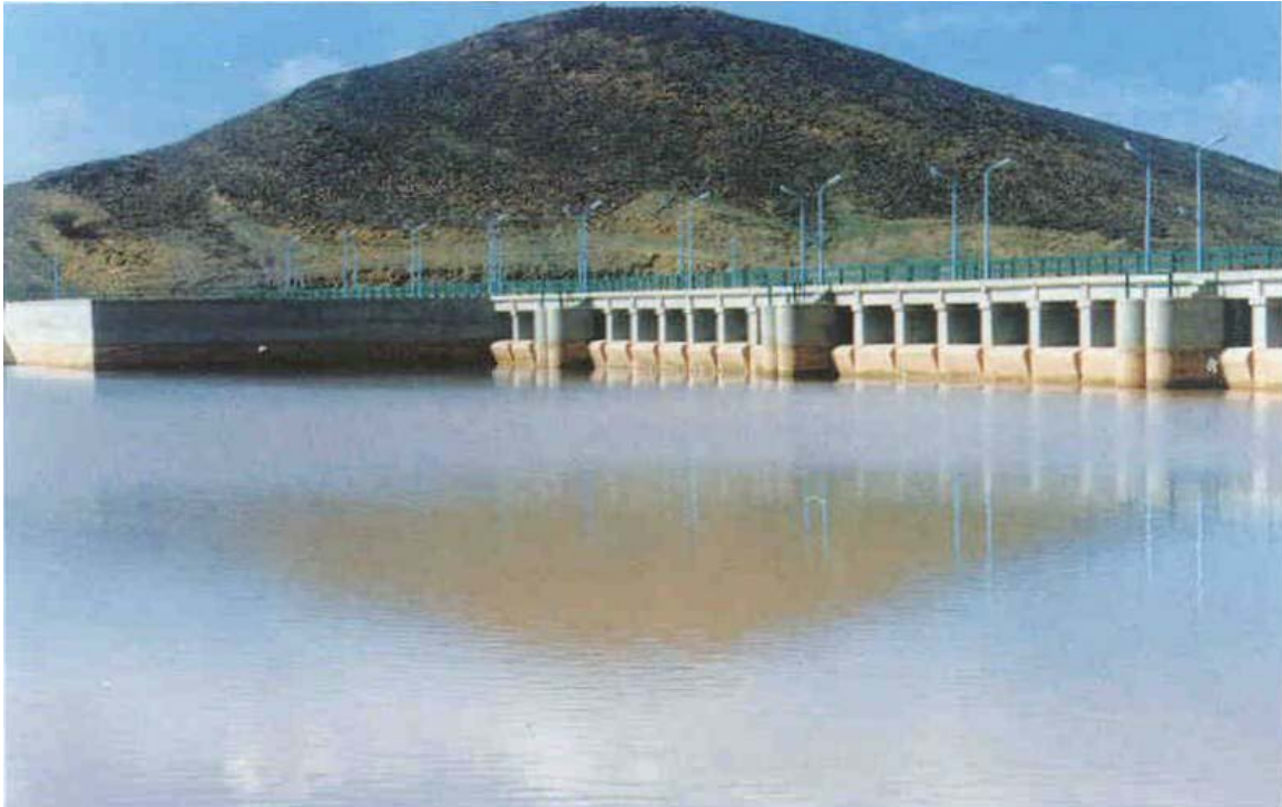
Figure 11g: Selected Pictures of Some Saudi Water Dams
